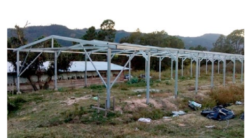
New chicken house under construction
